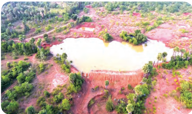
Fig.6.13 : Percolation tank
