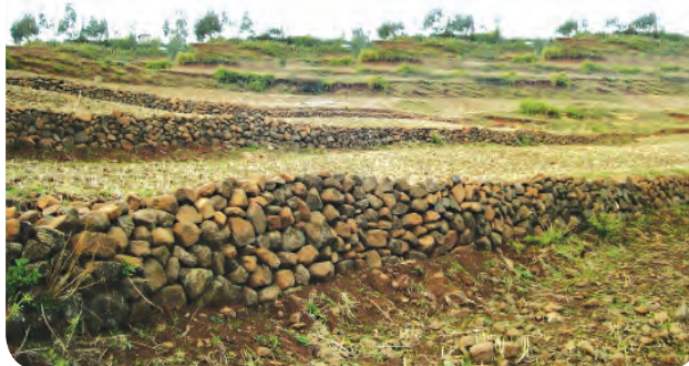
Fig. 6.10 : Stone contour bunding
