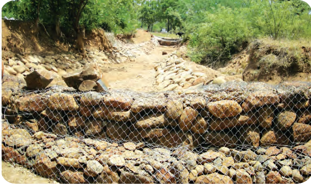
Fig. 6.12 : Gabion dam on stream
