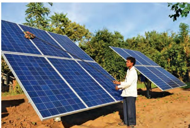
Solar panels - Non-Conventional Energy Source
