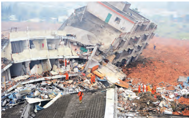
Effect of Earthquake
