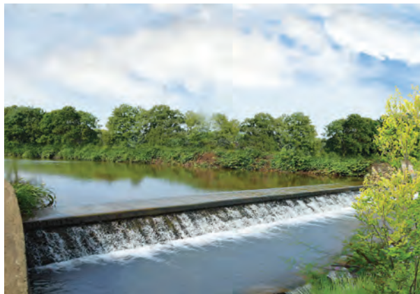
2.3.9 Concrete cement stream check dams
