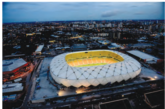
Figure 9.7 : Football Stadium at Manaus
