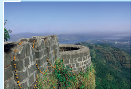
Figure 1.13 : Khadakwasla Dam as seen from Sinhagad
