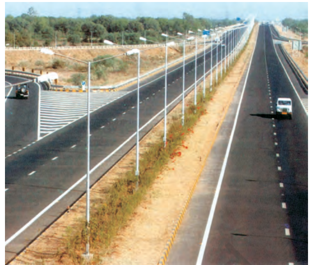
Fig. 7.2: Ahmedabad- Vadodara Expressway
