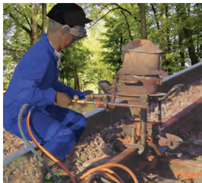
Figure 3.11 Thermit process for joining railway tracks
