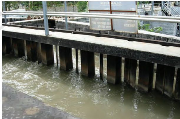
Fig. 13.4 Grit and sand removal tank
