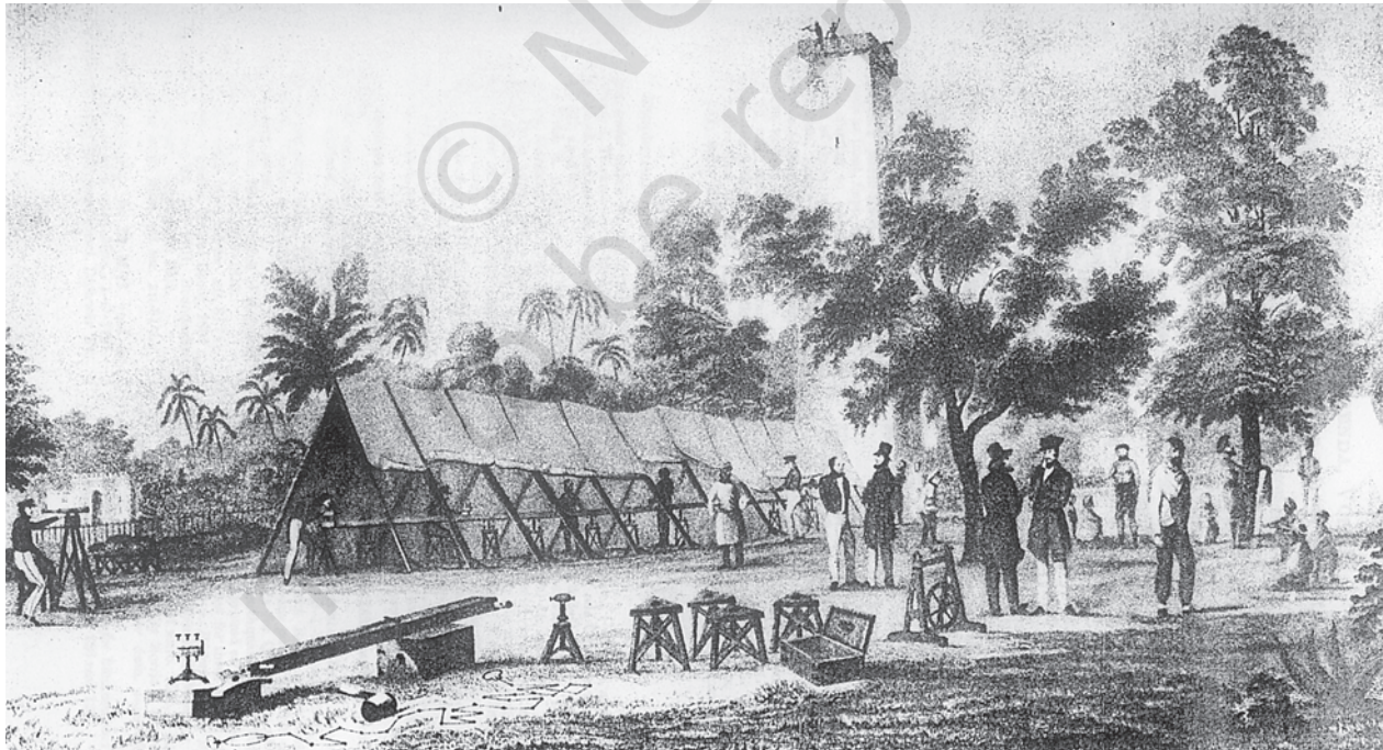
Fig. 6 – Mapping and survey operations in progress in Bengal, a drawing by James Prinsep, 1832 Note how all the instruments that were used in surveys are placed in the foreground to emphasise the scientific nature of the project.
